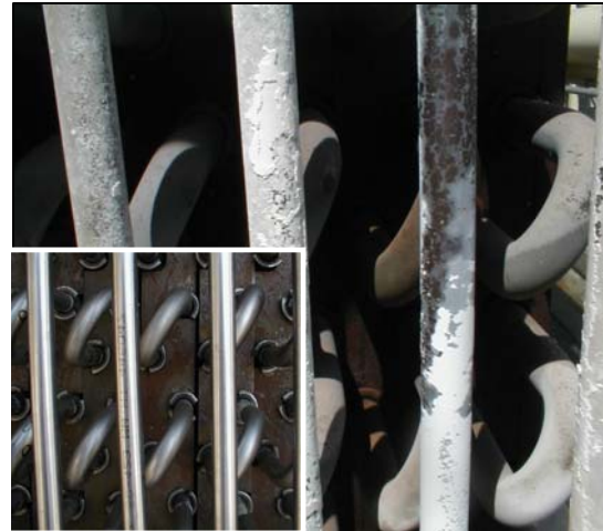
Figure 1. White Silicon Dioxide Deposits on Heat Recovery Steam Generators result in loss of 20% heating value and damage at $400K/yr.
